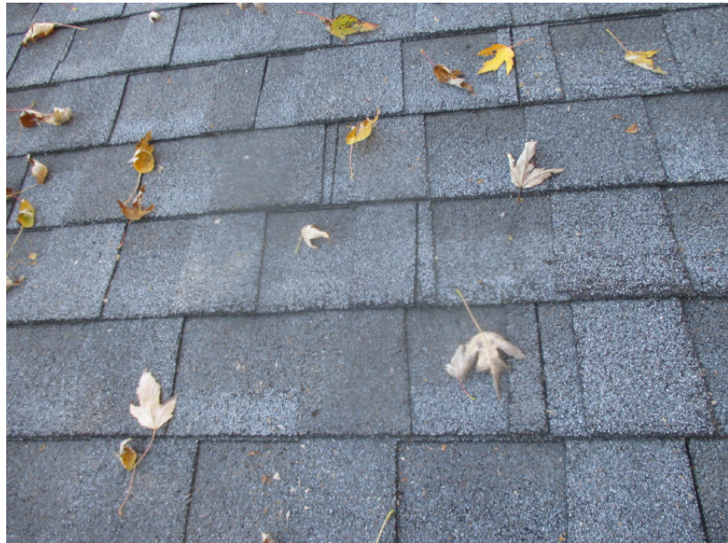
Note some shingle wear, but shingles intact and generally sound
