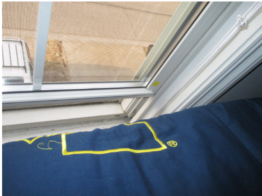
Sash being held in place by Inspector
