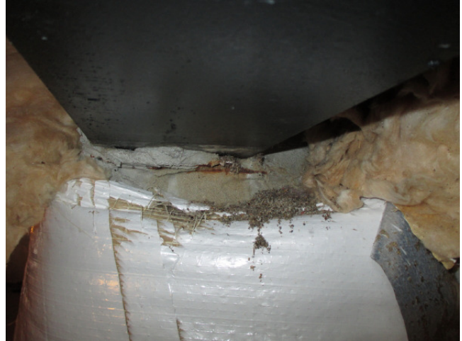
Area Client noticed leakage – note rust stain and sandy deposits consistent with insect activity
