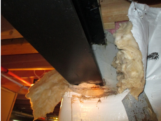
Area Client noticed leakage – note rust stain and sandy deposits consistent with insect activity
