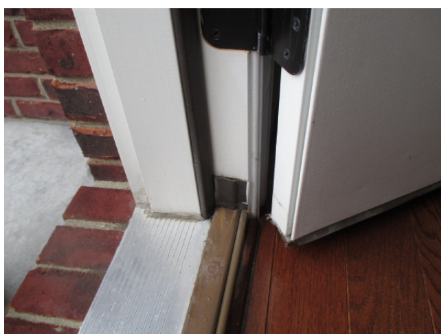
Door threshold through which water may enter, with sandy deposits like below
