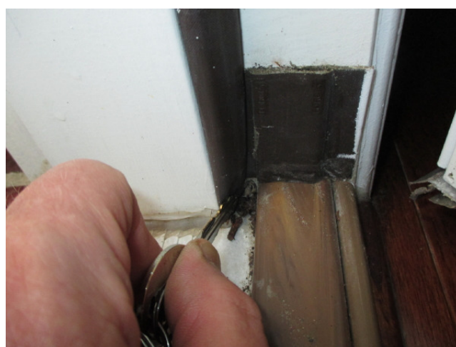
Door threshold through which water may enter, with sandy deposits like below
