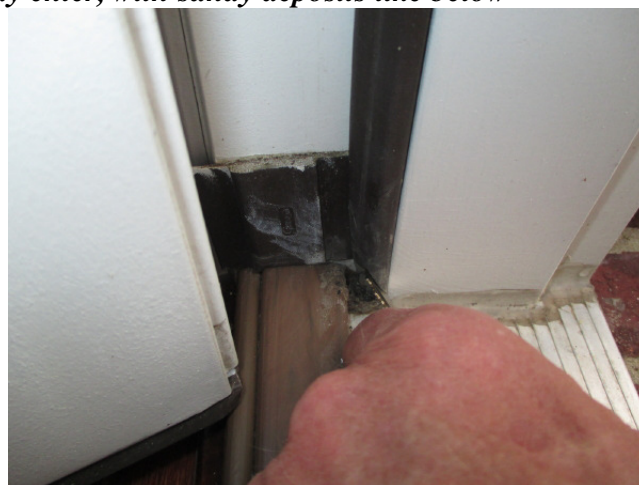
Door threshold through which water may enter, with sandy deposits like below
