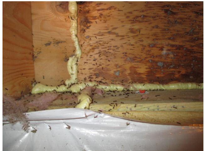
Wood below threshold – note stains, ant activity, and elevated moisture readings
