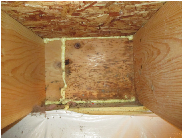
Wood below threshold – note stains, ant activity, and elevated moisture readings
