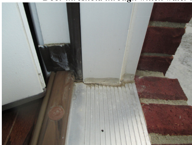
Door threshold through which water may enter, with sandy deposits like below
